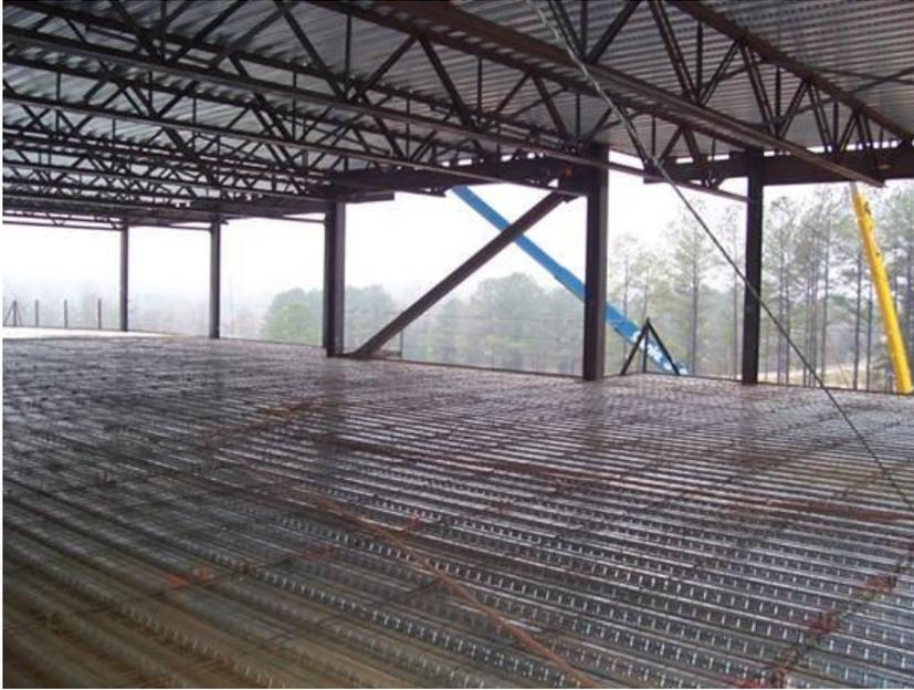
Steel deck functions as the primary supporting surface for roofing materials and as form and/or positive reinforcement for concrete floor slabs.
